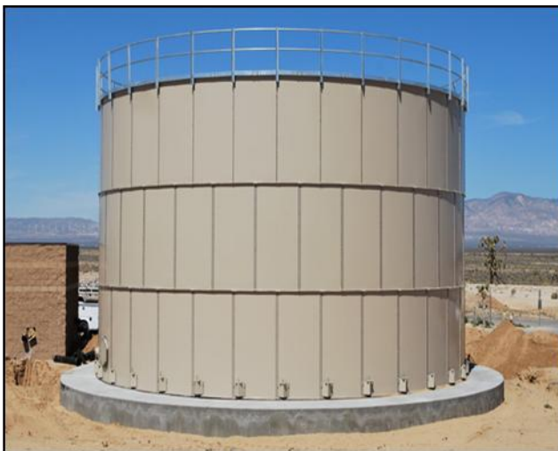
Figure 4-15 Treated effluent storage tank
